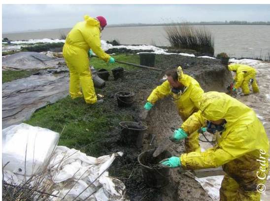
Manual clean-up site
