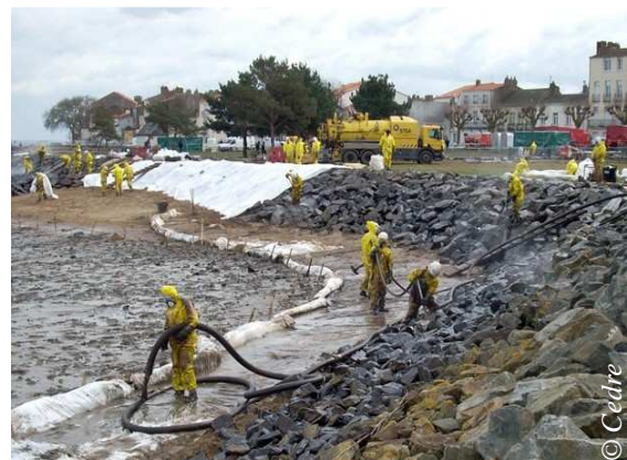
Mechanical clean-up on riprap
