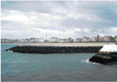
3. Manmade structure (ESI 2)
